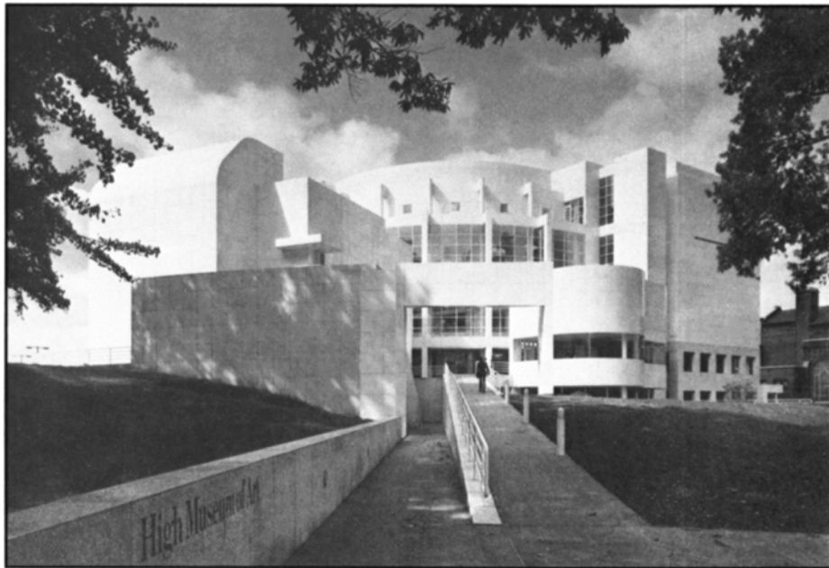
23 Richard Meier, High Museum of Art, Atlanta, view from entrance ramp toward atrium, 1983
